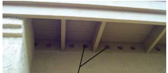
Trapped heat and gases could enter through the vent holes in these exposed eaves. (FEMA)
