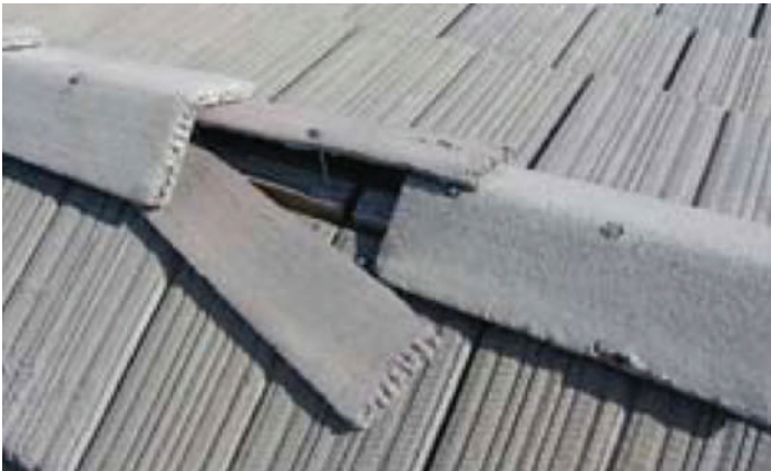
Displaced tiles, no matter how good, will allow ember entry. (FEMA)
